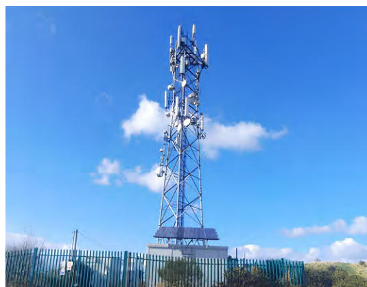
Solar powering a base station at Tullow Hill in Ireland
